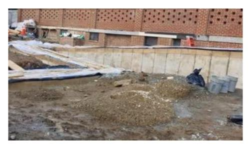
During January, the concrete work for the ramp was completed. The rails for the ramp have been ordered and will be installed as soon as they arrive. Rocks have been delivered to fill in space between the ramp and the wall. Work is three-quarters done on the reinforcement of the column supporting the back portion of the building. Landscape work is scheduled for the spring.
